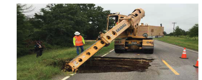
Sink hole in the road being fixed by a work crew.
