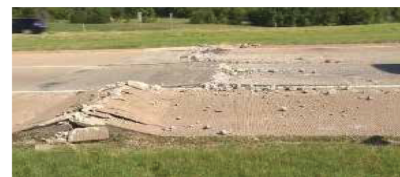
Road buckling from extreme heat on US Highway 75 southbound in Denison, Texas. July 2016. Source: KXII.
