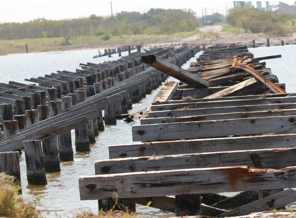
Washed out beams from the old railroad bridge crossing from Oso Bay to Flour Bluff, at the location of the new Trestle Bridge. Source: Corpus Christi Parks and Recreation, Caller-Times Contributed
