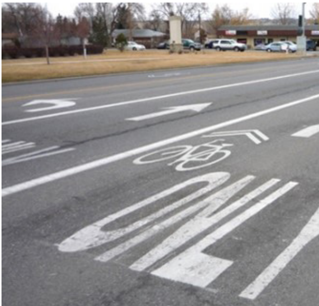
Combined Bike Lane/Turn Lane Places a suggested bike lane within the inside portion of a dedicated motor vehicle turn lane. Shared lane markings or conventional bicycle stencils with a dashed line can delineate the space for bicyclists and motorists within the shared lane or indicate the intended path for through bicyclists.
