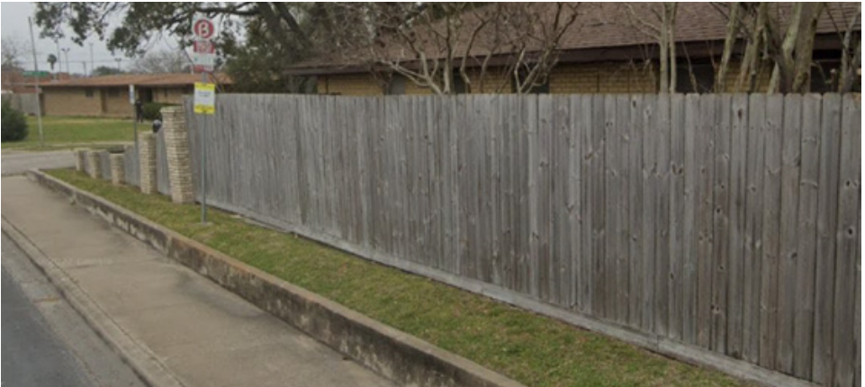
Example of an inaccessible bus stop in Corpus Christi. The pad at the bus stop at Airline Road at Monette Drive does not have the required depth (96”) to be ADA-compliant. (Source: Google Street View)
