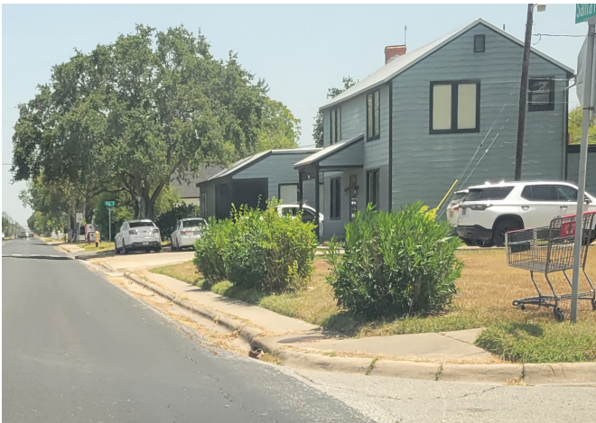
Sidewalk at curb-face with insufficient buffer from traffic on Santa Fe Street, Corpus Christi, TX
