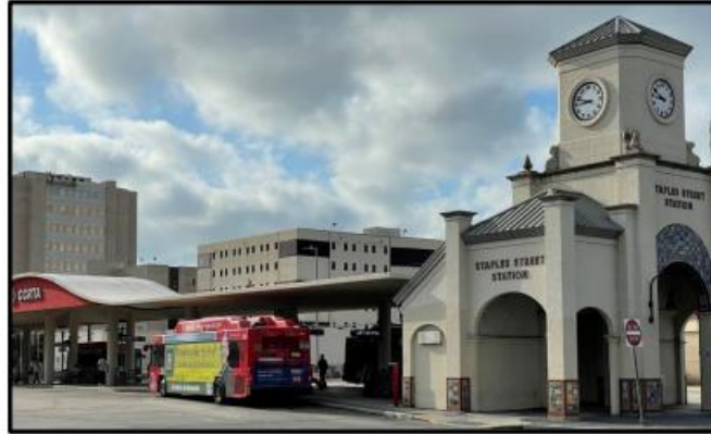
Figure 8 - Staples Street Station
