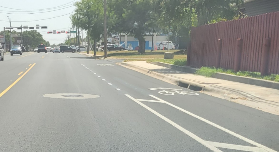
Doddridge Street, Corpus Christi, TX (Source: FNI)
