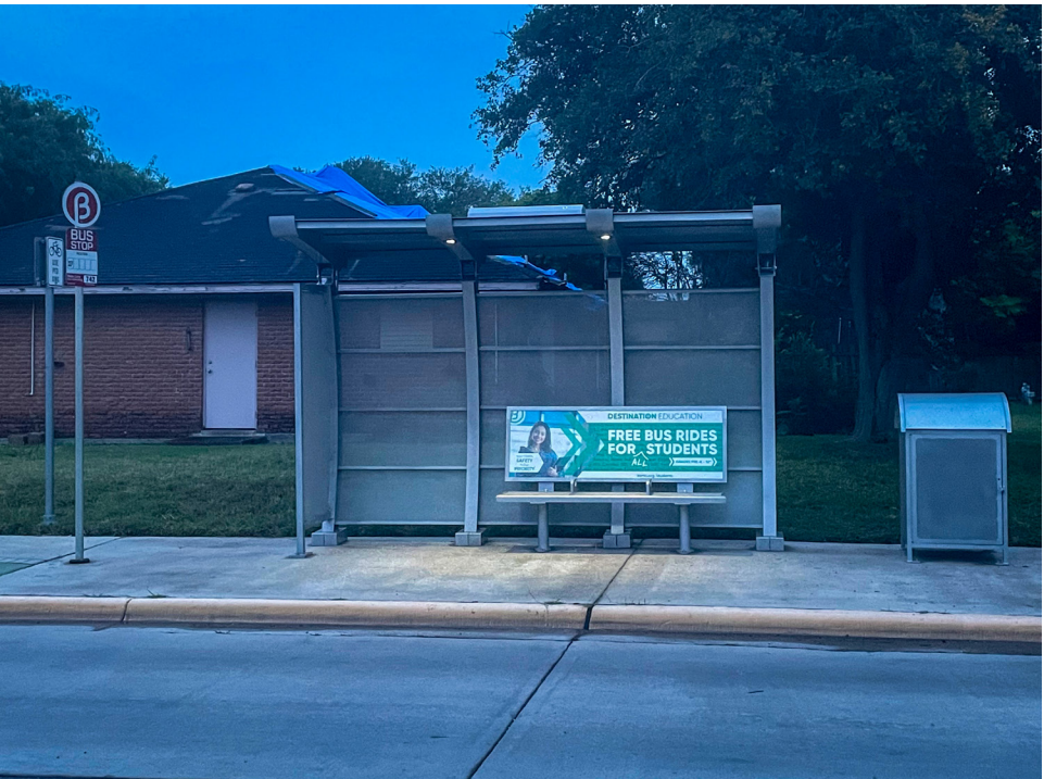
ADA-compliant bus stop in Corpus Christi.
