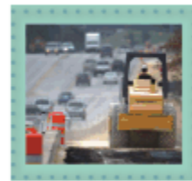
Freeway Widening $6.1 million per lane mile
