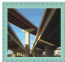
Overpass $5.8 million per lane mile
